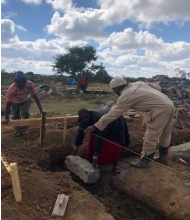
Construction of a local well
